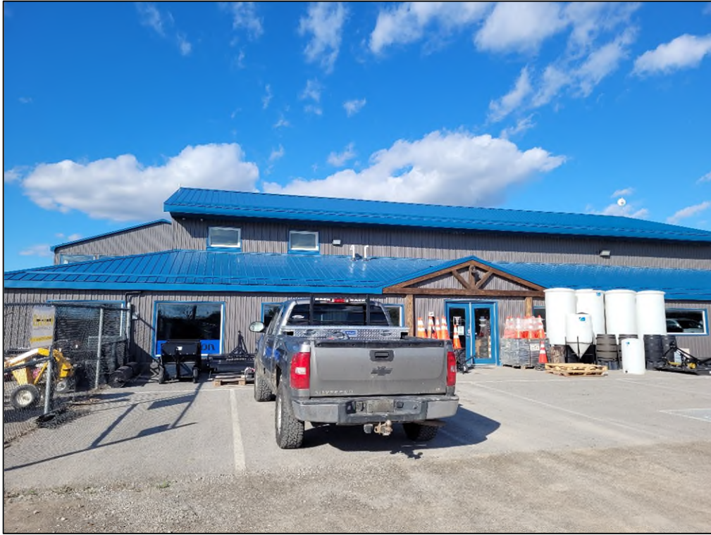
Figure 2 - Existing Office and Retail Space (5377 Elcho Road)
