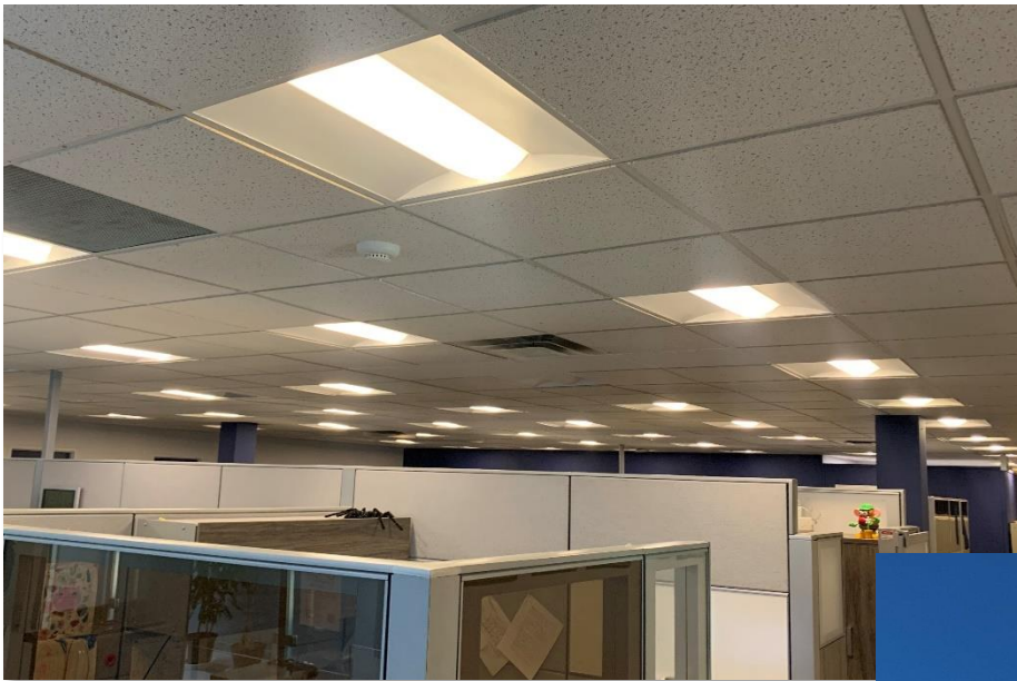
Figure 2.1 Town Hall Lighting Upgrade
