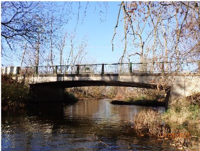
Photograph No. 2: 0433: East elevation.
