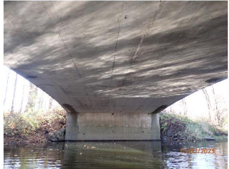
Photograph No. 3: 0442: Underside of the structure looking south.
