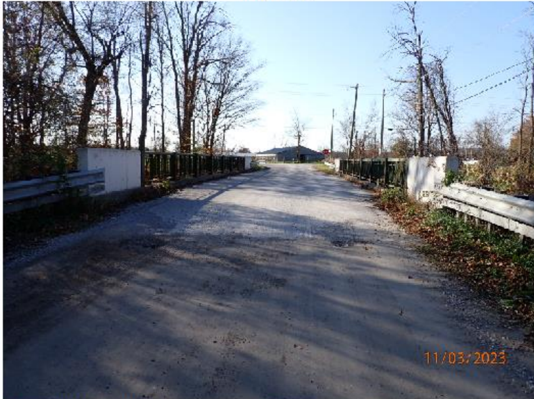
Photograph No. 1: 0362: Roadway over the structure looking south.
